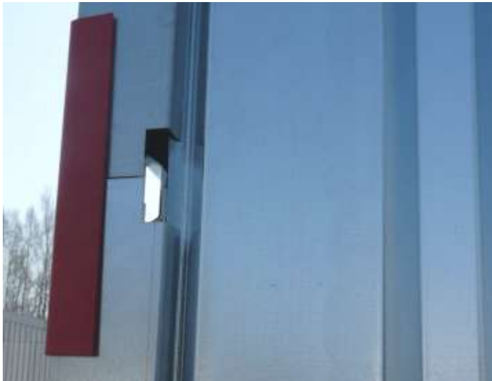
Picture no. 13 Opening before covering
